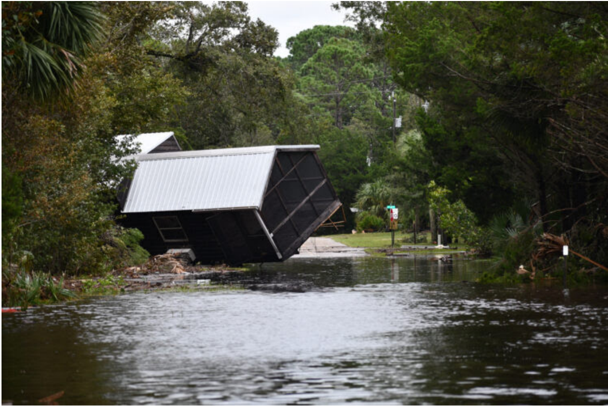
Image of damage after Hurricane Idalia by USFWS
