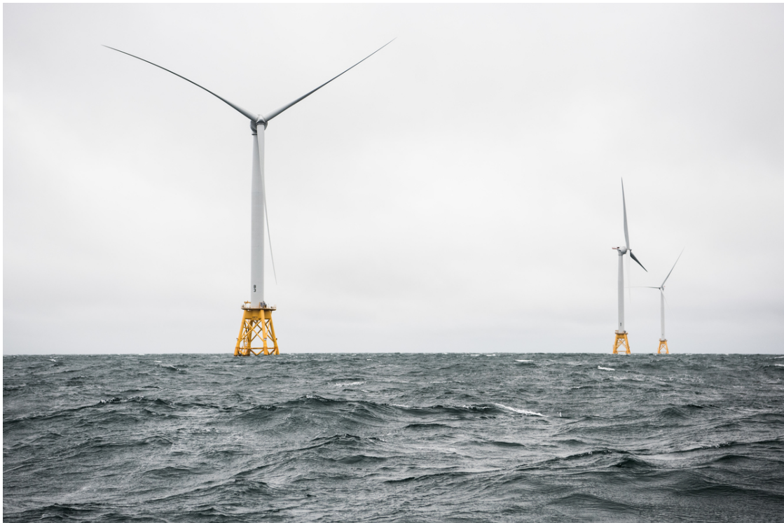
Photo: Dennis Shroeder/National Renewable Energy Laboratory
