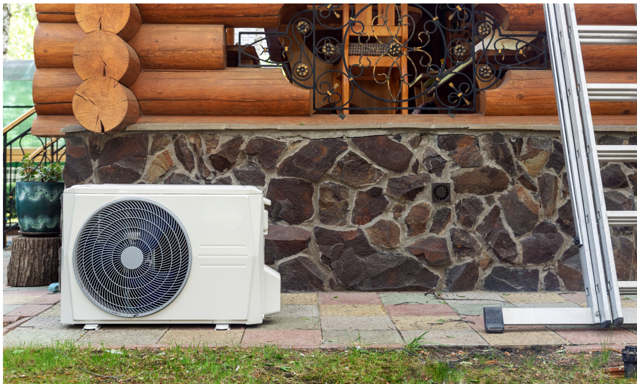
Heat Pump HVAC External Compressor Unit
