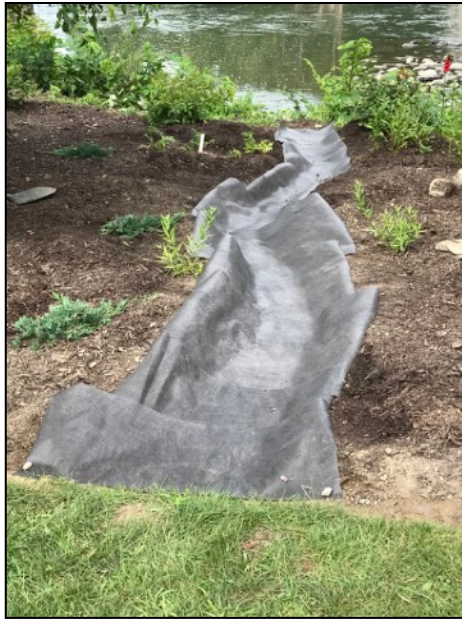
Drainage is needed
