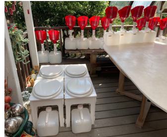
Waterless unisex “Cubie” urinals and “Pee-Toilets”
