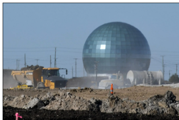
Site preparation began in 2023 at the site of the new Microsoft data center campus in Mount Pleasant. Originally encompassing 315 acres, Microsoft’s local footprint is expanding to 1,345 acres for an expanded campus, in the area originally purchased by the village for Foxconn. Foxconn’s data center globe is in the background. Phase 1 is scheduled to open in 2026. Photo by Mark Hertzberg for Racine County Eye
