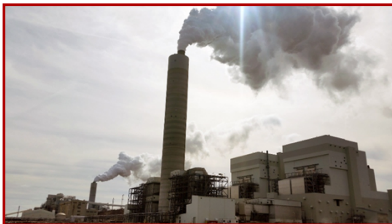
We Energies' coal-fired Oak Creek power plant. Photo by Chuck Quirnbach/wpr.org
