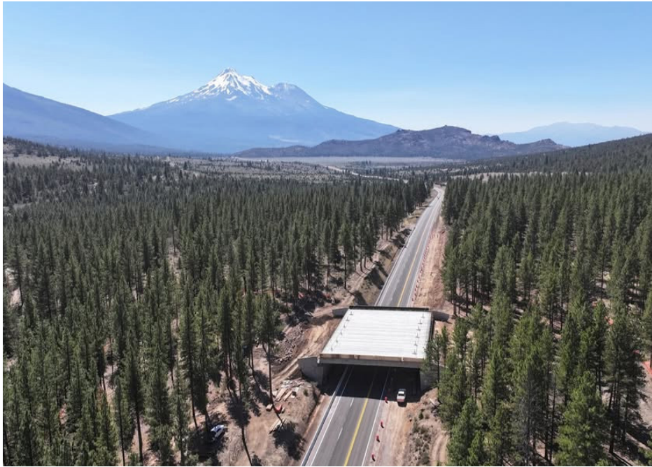
Drone photo shows the newly completed highway overcrossing in Siskiyou County
