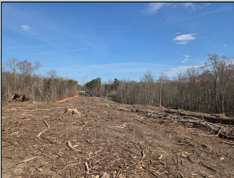
March 30th Tree cutting along Eskimo Hill Rd.
