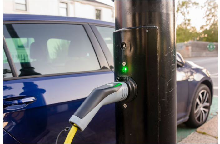
Electric car being charged from a charging point on a street light post. Stephen Barnes
