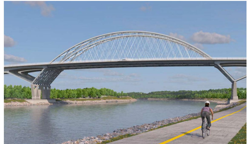
Bridge Type – Twin Network Tied Arch
