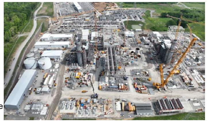
TVA began construction on the Cumberland Gas Plant, located adjacent to the Cumberland Fossil Plant, in 2023. The facility is expected to be in operation by the end of 2026.
