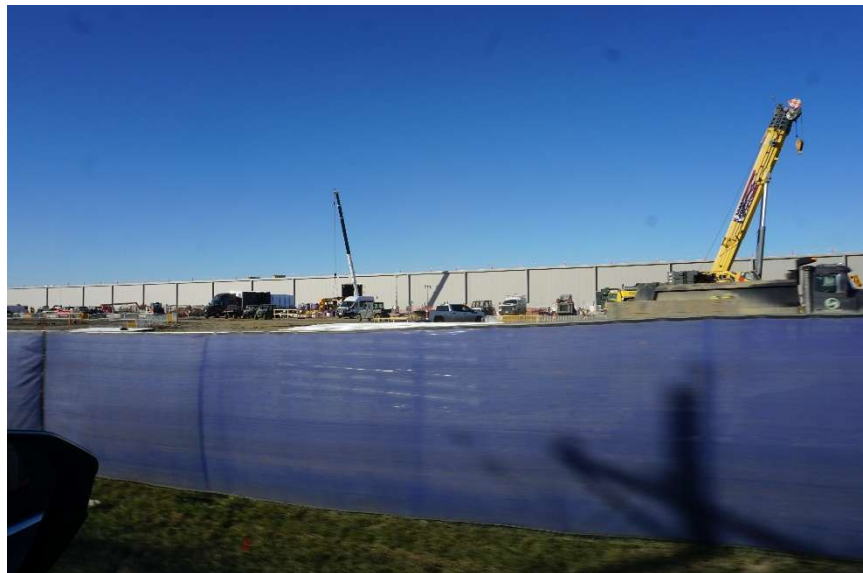
A data center under construction in Cedar Rapids, Iowa. Photo by Pam Mackey Taylor
