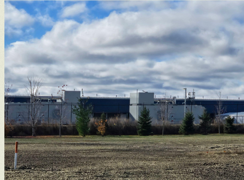
Photo of data center by Jess Mazour
