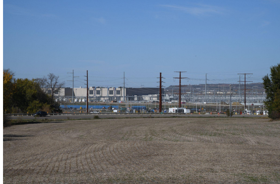
Photo of data center in Council Bluffs, by Tom Reardon
