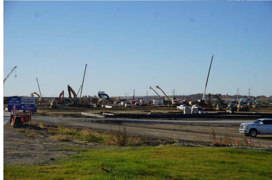
Photo of data center construction in Cedar Rapids, by Pam Mackey Taylor
