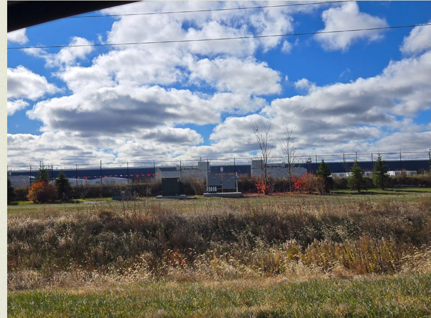
Photo of a data center by Jess Mazour
