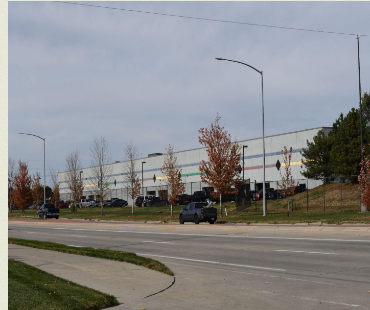
Photo of a data center in Council Bluffs by Tom Reardon
