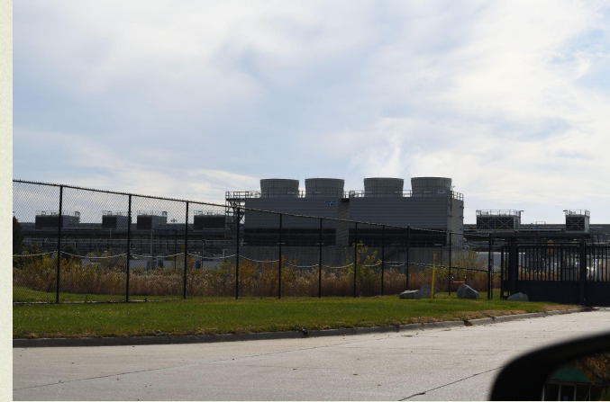
Photo of a data center in Council Bluffs by Tom Reardon
