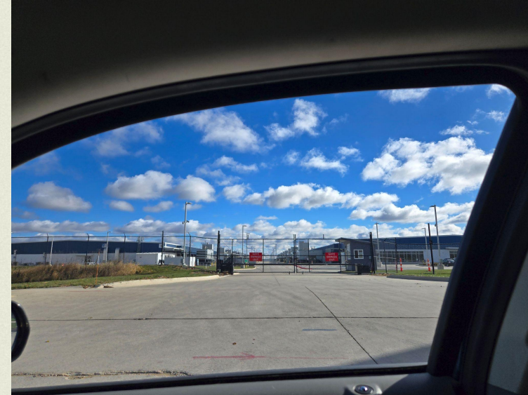
Photo of data center by Jess Mazour
