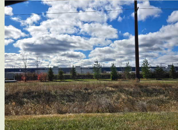
Photo of data center by Jess Mazour
