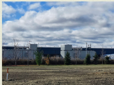
Photo of data center by Jess Mazour
