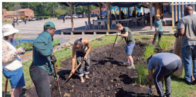
Stormwater Specialist Training class gaining hands on experience installing a rain garden at St. Suzanne Cody Rouge Community Re-
