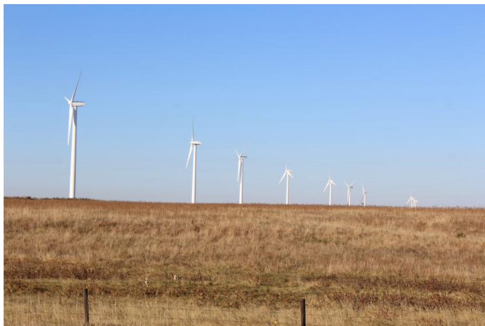
Greensburg's 10 turbines, at 1.25 MW each.
