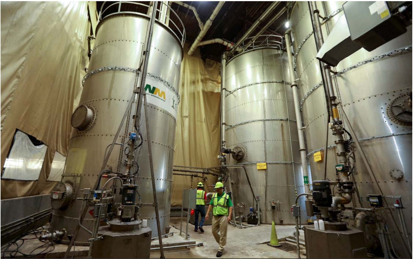
Workers at the Waste Management facility in North Brooklyn, N.Y., process sewage into bio-slurry for conversion into methane gas.
