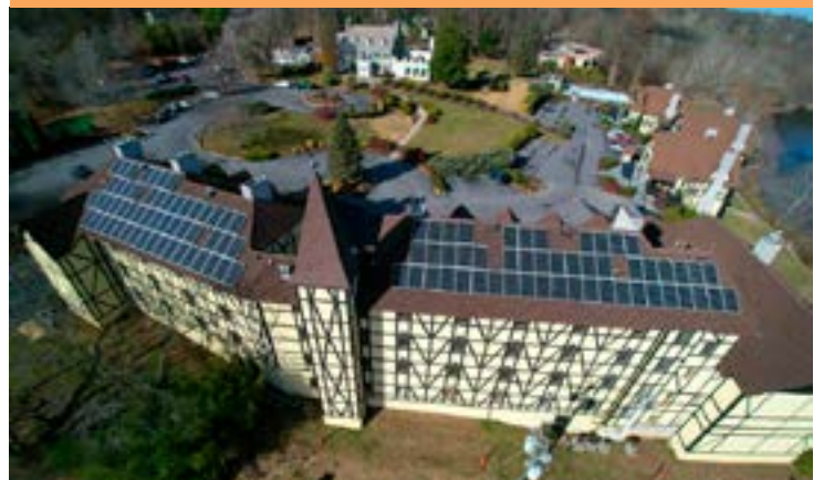
SOLAR AT THE BAVARIAN INN, SHEPHERDSTOWN, WV IMAGE CREDIT: MOUNTAIN VIEW SOLAR
