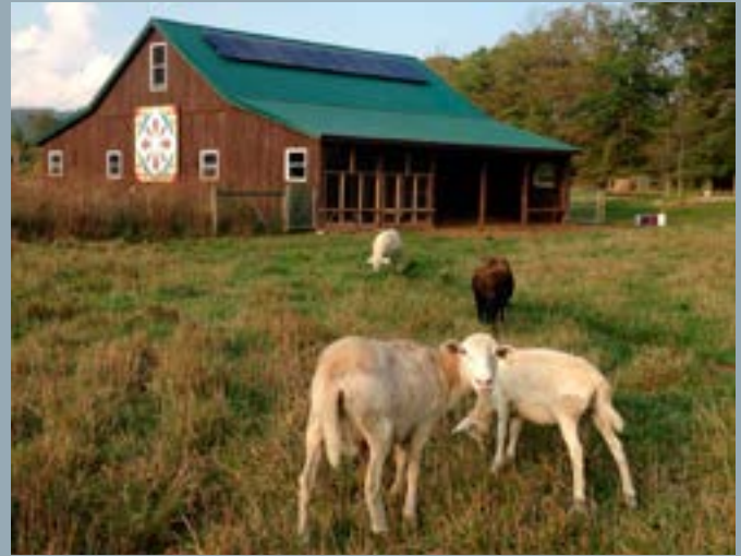
SOLAR INSTALLATION ON THE REESE BARN, IMAGE CREDIT: TIM REESE
