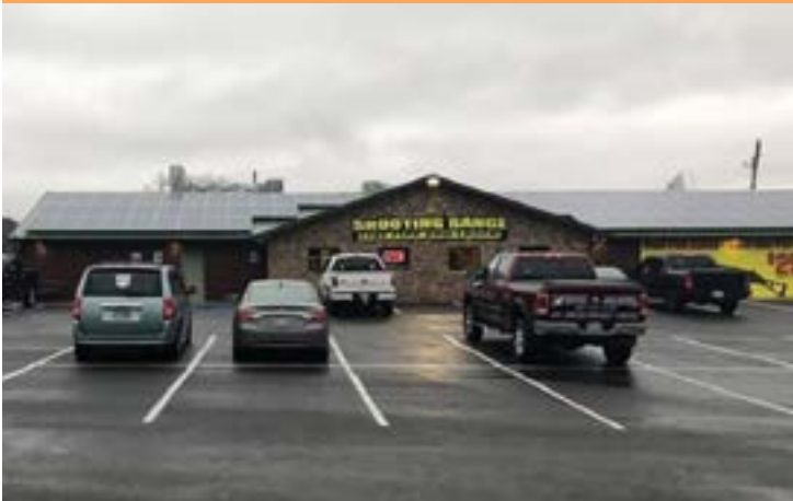
CROSS HAIRS SOLAR ARRAY, IMAGE CREDIT: BIG D ELECTRIC
