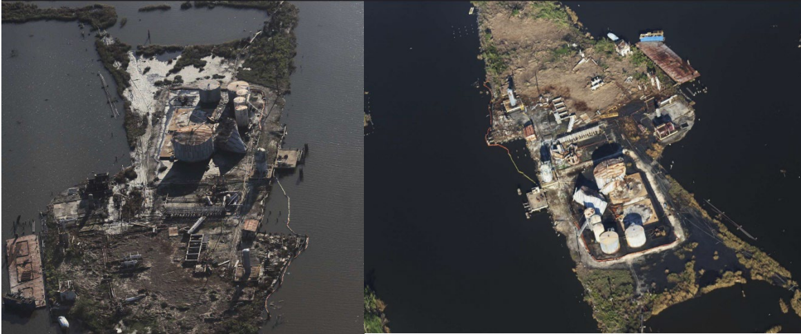
Figures 8 a and b. photos of damage to an oil and gas facility baywards of the LNG site during the passage of Hurricane Ida.
