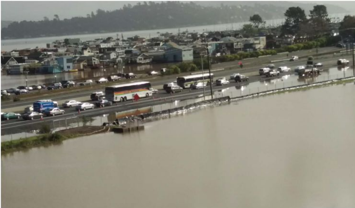
Figure 3: February 2017 Flooding – looking southeast over detention basin to US 101 offramp
