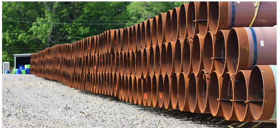
Staging area in Ohio for construction of the Rover gas pipeline. Ted Auch. May 3, 2017. Provided by FracTracker Alliance, fractracker.org/photos .
