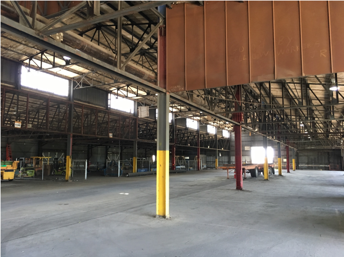
Photograph 3 View from inside Wharf 8 building looking southeast
