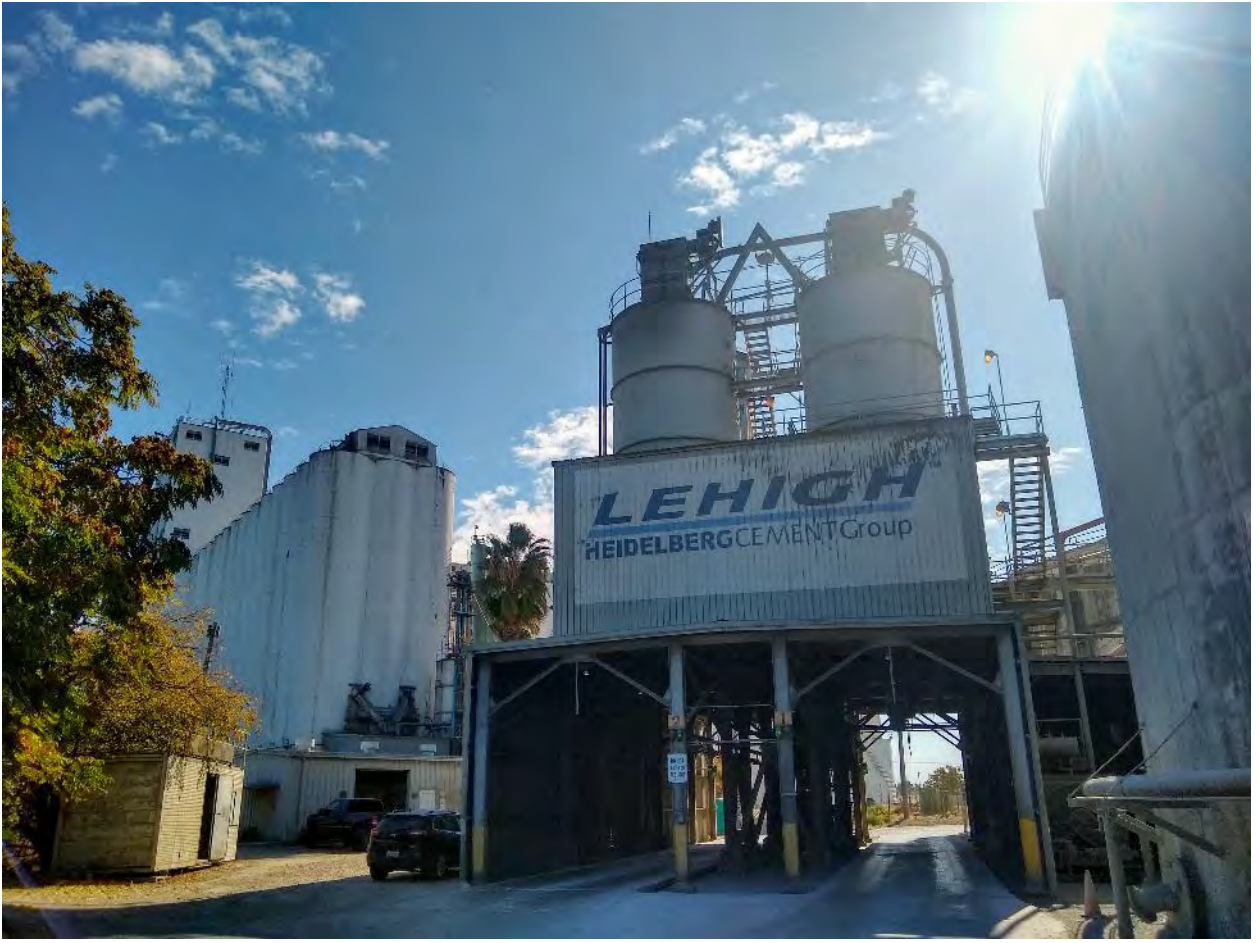
Photograph 3 Existing Truck Loading Stations
