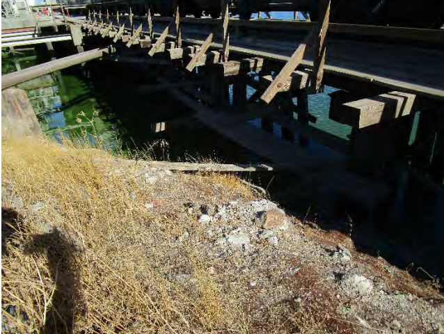
Overview of trestle; View: North; Date: 09/26/19; Acc. #: 19-0016-2288
