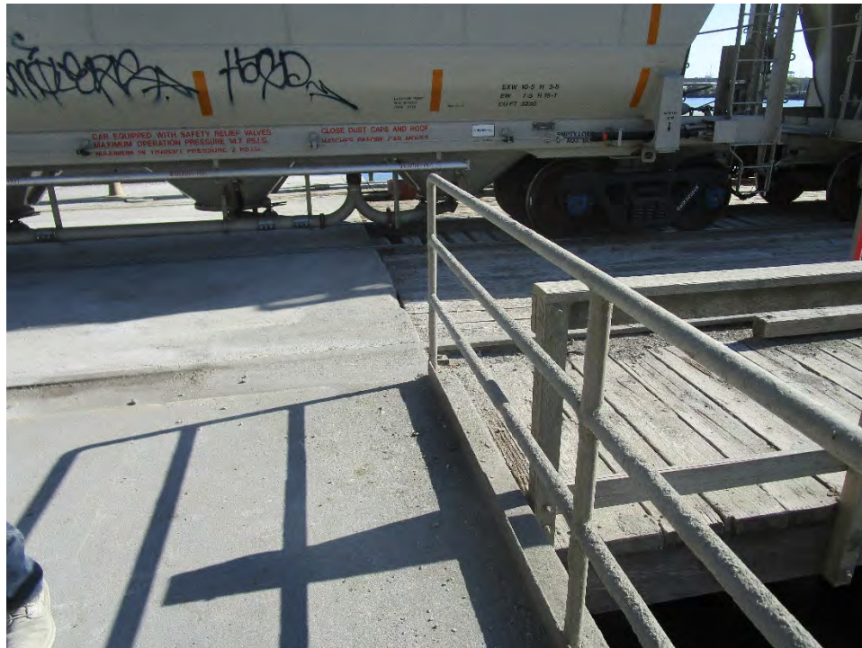
Berth 2 and rail trestle junction; View: East; Date: 09/26/19; Acc. #: 19-0016-2280
