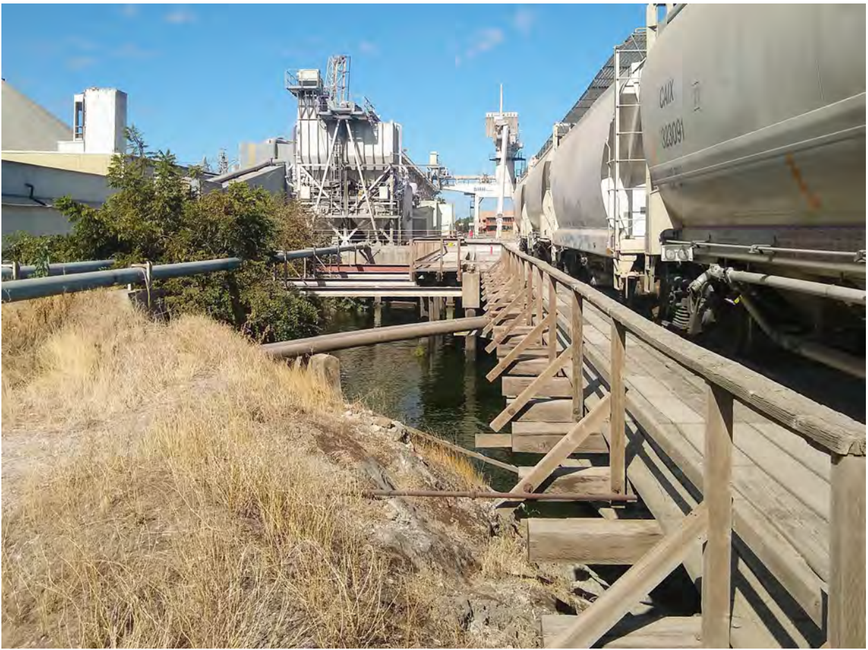
Photograph 2 Existing Wooden Rail Trestle with Empty Rail Cars
