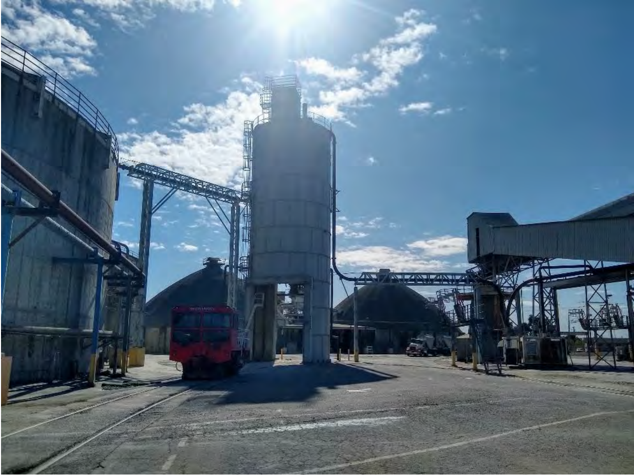
Photograph 5 Existing Rail Car Loadout
