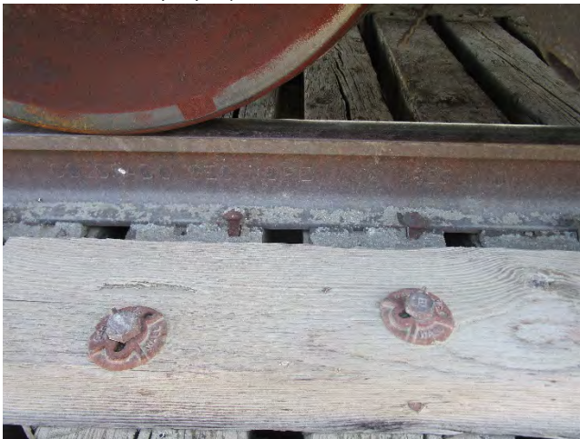
Rail section with 1929 date stamp; View: East; Date: 09/26/19; Acc. #: 19-0016-2293
