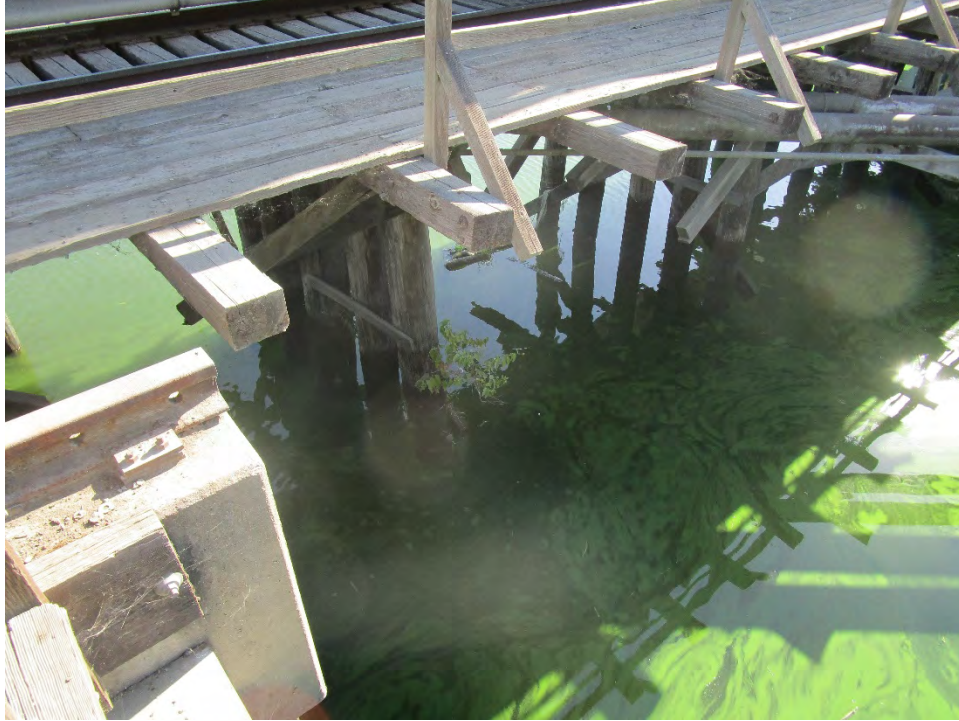
Underside of trestle; View: East; Date: 09/26/19; Acc. #: 19-0016-2285
