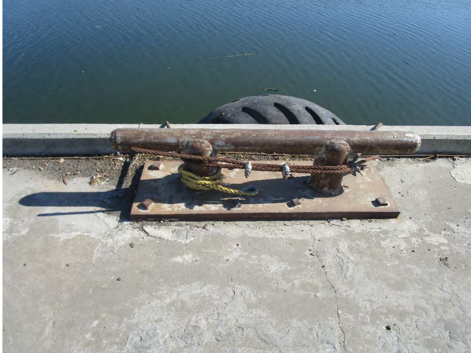
Berth 2 mooring; View: Detail; Date: 09/26/19; Acc. #: 19-0016-2301
