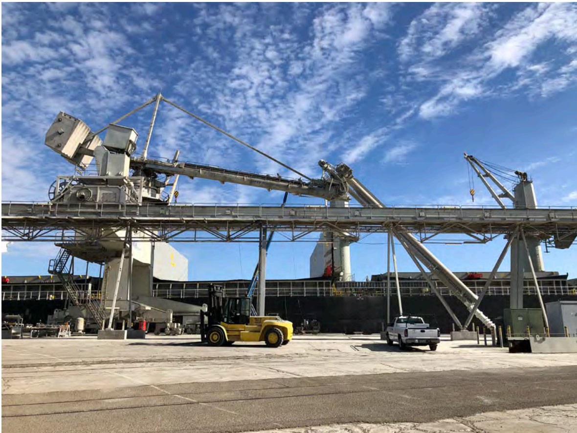
Photograph 1 Existing Bulk Cementitious Material Terminal
