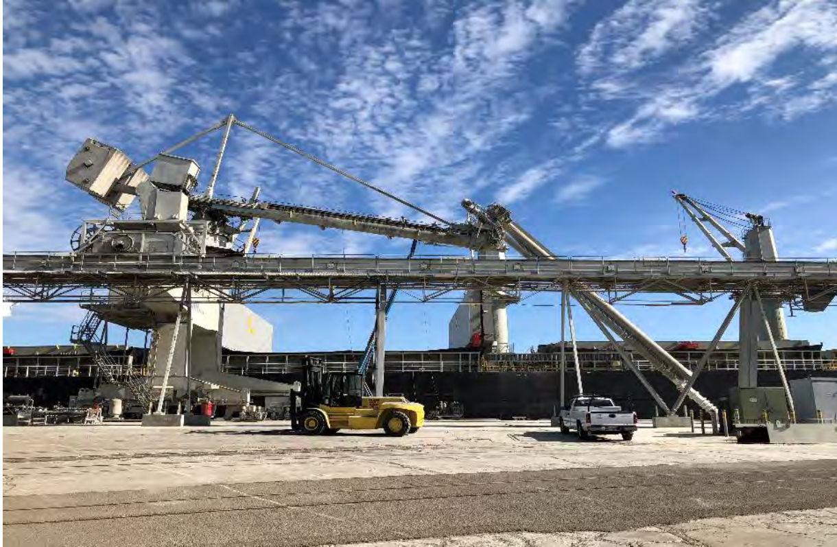
Photograph 1 Existing Ship Unloader
