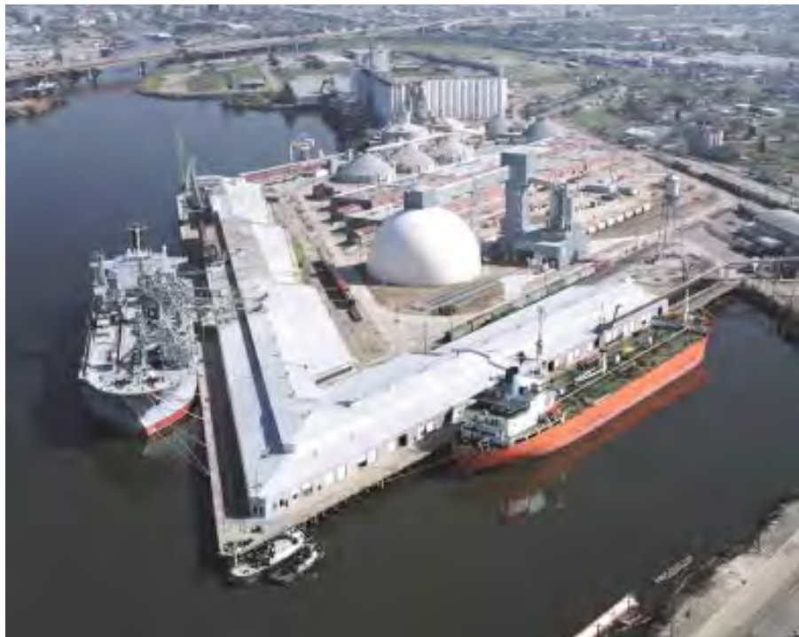
Port of Stockton East; View: East; Date: 2002; Courtesy: Port of Stockton
