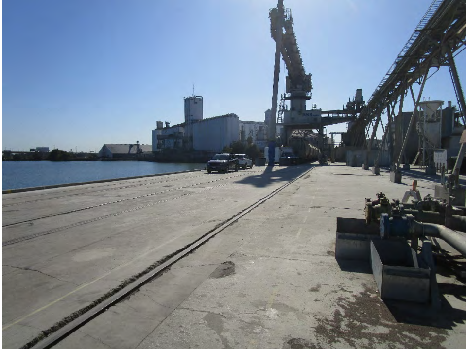
Overview of Berth 2 at Port of Stockton Eastern Complex; View: Southeast; Date: 09/26/19; Acc. #: 19-0016-2305
