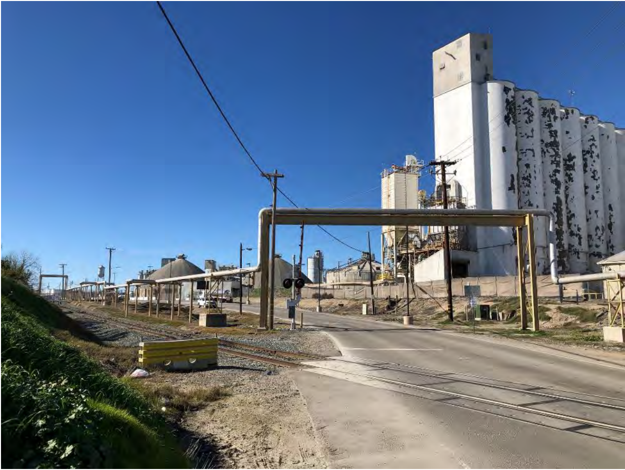
Photograph 7 View of Lehigh Terminal from Harbor Street (Southeast of the Project Site)
