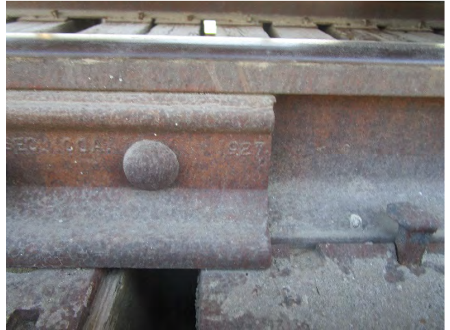
Fishplate with 1927 date stamp; View: Detail; Date: 09/26/19; Acc. #: 19-0016-2292
