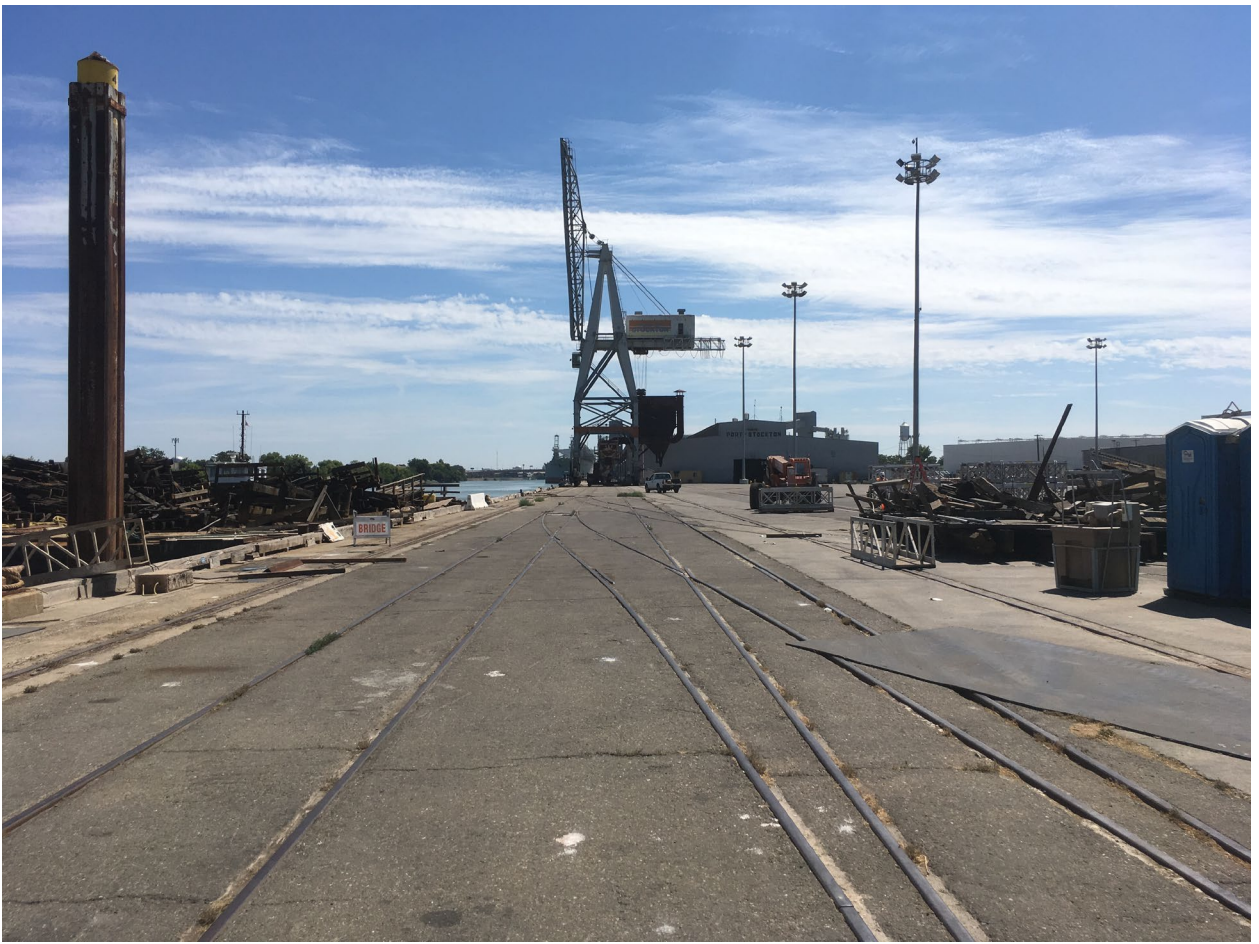
Photograph 3 Dock 10/11 asphalt and concrete deck
