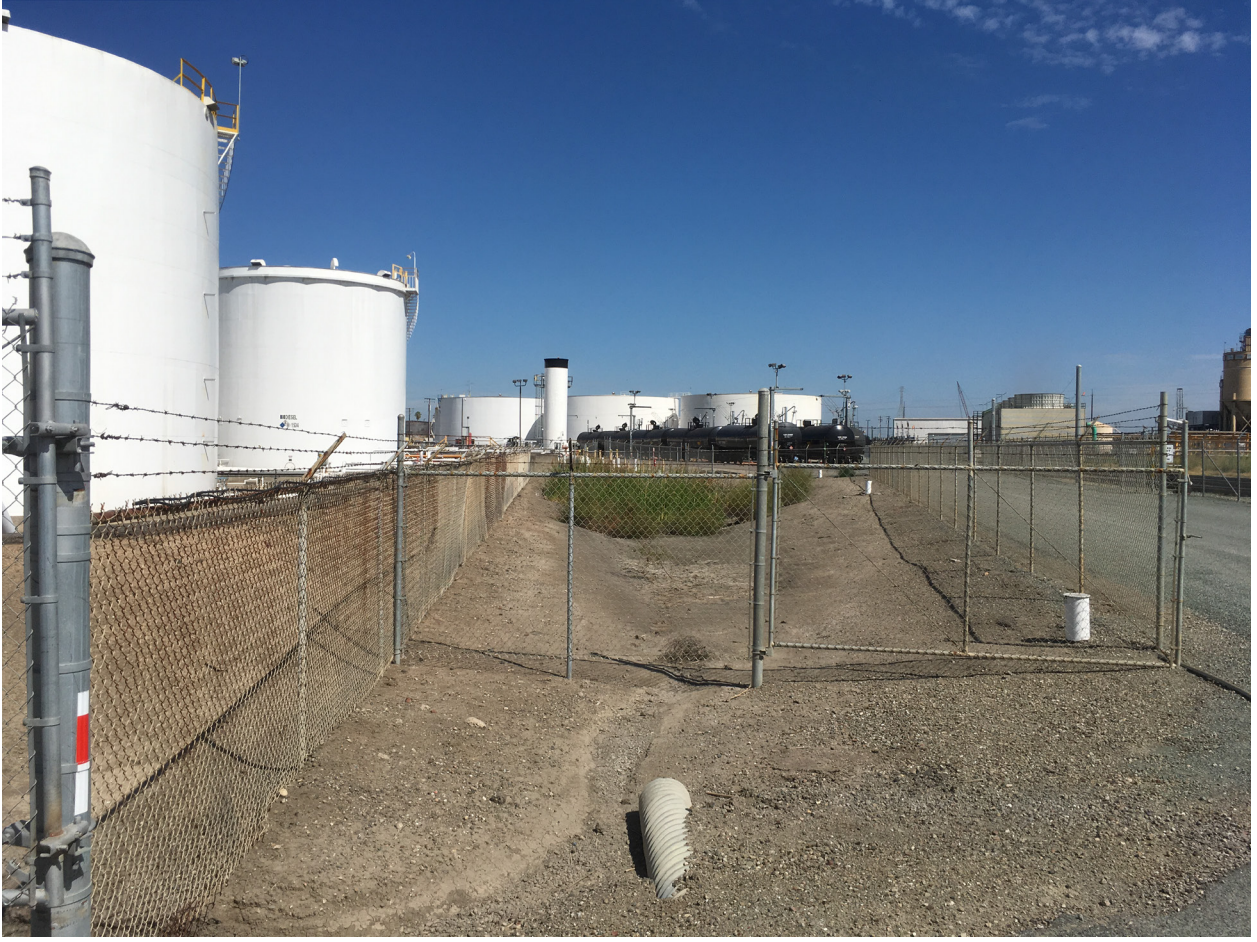
Photograph 2 NuStar facility storm drain and pond system
