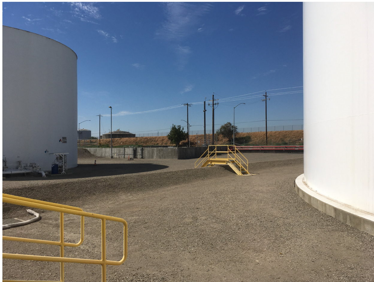
Photograph 3 Tanks and containment berm at the NuStar facility
