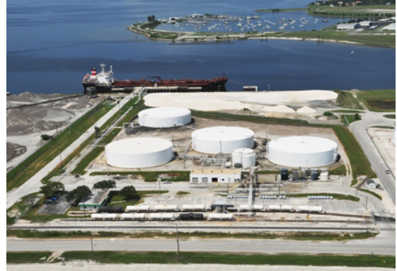
< SATCO Tank Terminal / Tampa, Florida, US>
