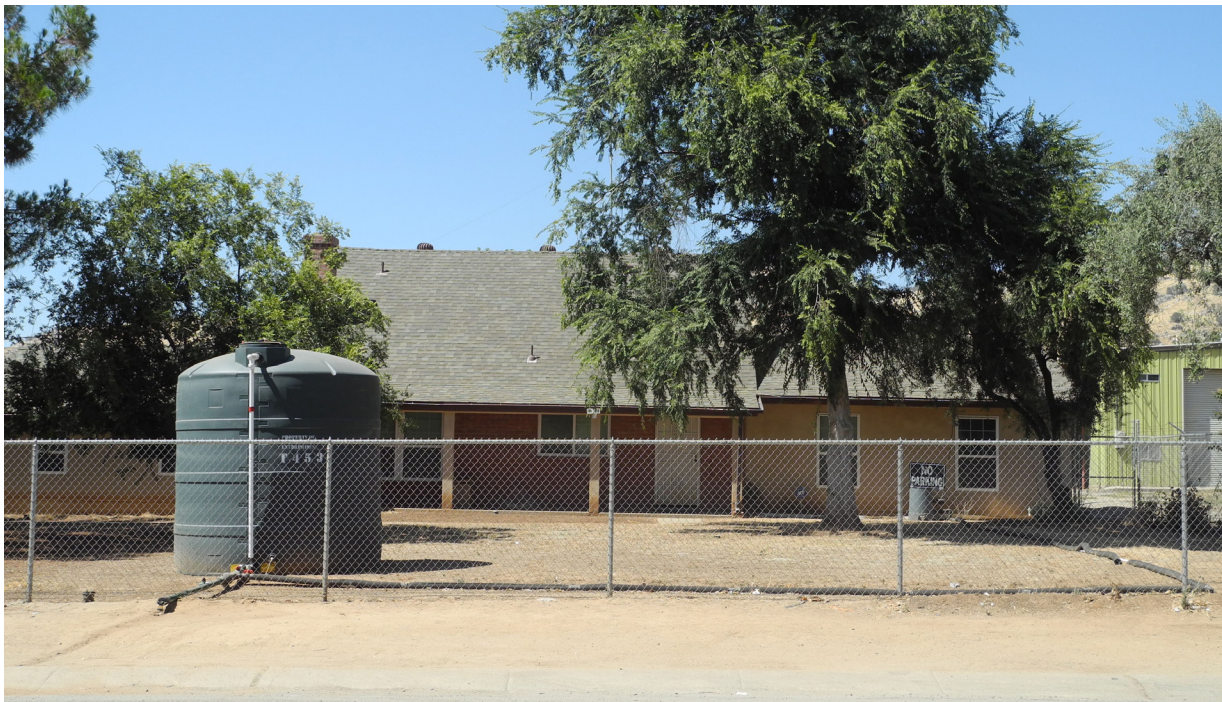
House receiving water from a temporary emergency tank due to dry groundwater well.
