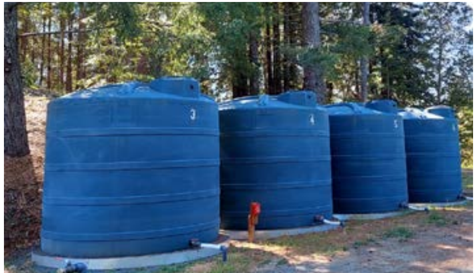
Four, 5,000-gallon water tanks were installed on a neighboring property as additional supply for fires and drought. Photo: Tom Roth.
