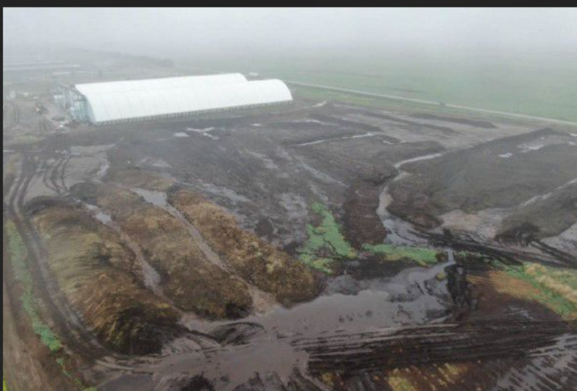
An estimated 250,000 cubic yards of pesticide-laden wet cake — a volume of solid byproduct that would cover the area of a football field at a depth of 150 feet — is stockpiled at three sites on AltEn's property.
