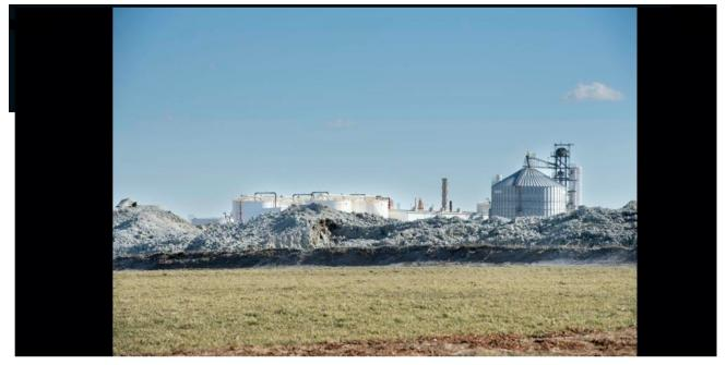
In mid-February, Posi-Shell, a combination of cement, clay and polyester fibers, was applied to a pile of wet cake and sludge produced by the AltEn ethanol plant near Mead.
