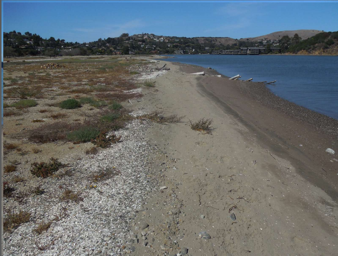
Dec 5, 2012 post construction Apr 16, 2013 post significant southern storms
