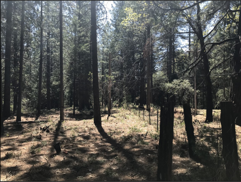
Fuels reduction work along Vilas Rd. in Cohasset funded by a California Climate Initiative Grant
