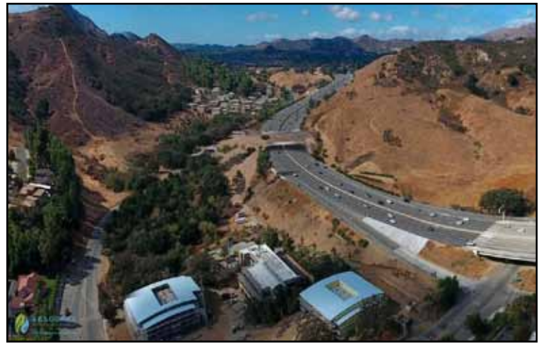
Liberty Canyon Wildlife Crossing will break ground on Earth Day, April 22. This is a Virtual-Image of how it will look. There will be on- or near-site viewing and live streamed video. Purpose is to provide a safe and sustainable passage for wildlife (and drivers) across US-101 in the City of Agoura Hills and allows for exchange of genetic material. It is a public-private partnership that has leveraged the expertise and leadership of dozens of organizations and institutions.
