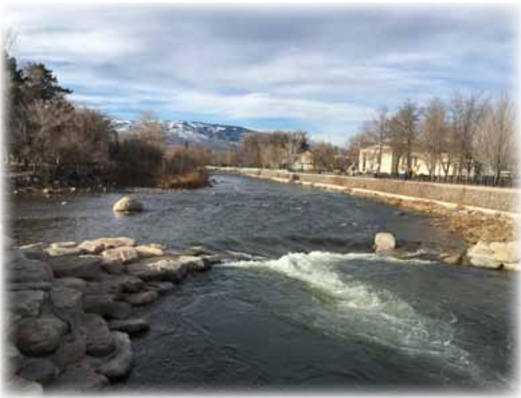
“Green flood control” that recharges storm water seems to be a no-brainer and already demonstrated here along the Truckee River. So why can’t we do it for the Santa Clara River? (Photo contributed)
