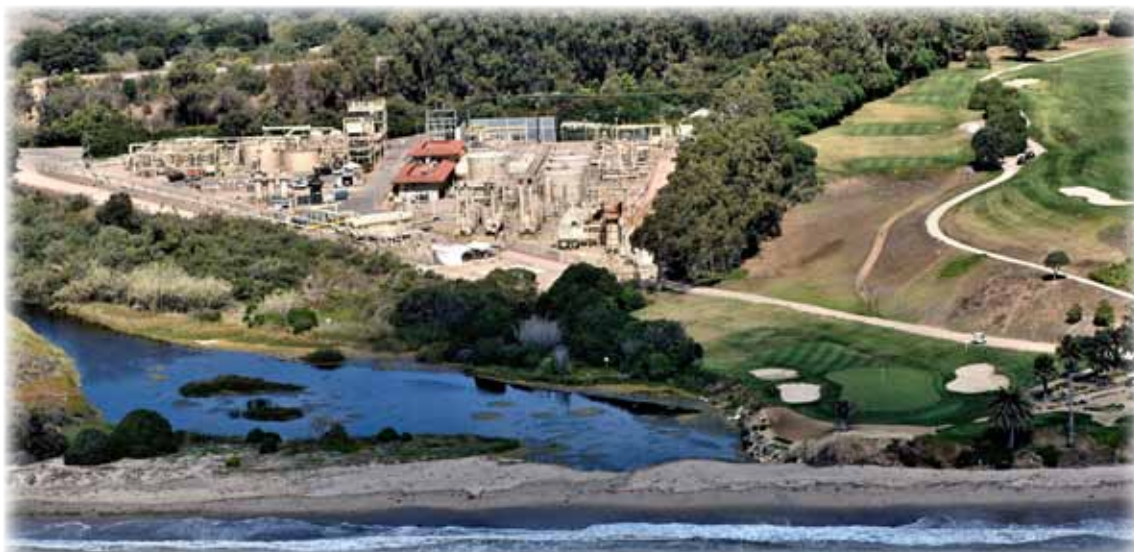
Venoco's Oil Processing Facility for Platform Holly that will now be dismantled. This aerial is part of the California Coastal Records Project which entails keeping a photographic record of whole coast. Read more info at: www.Californiacoastline.org (Copyright © 2002-2017 Kenneth & Gabrielle Adelman)
