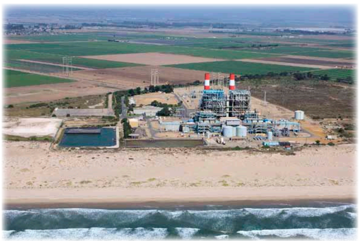
Many Oxnard residents have had enough of industrial uses on its beaches, but instead of being phased out, SoCal Edison wants to put in a new peaker plant; albeit to replace two older ones. Shown is an existing plant on Ormond Beach. (Photo Copyright © 2002-2017 Kenneth & Gabrielle Adelman Coastal Project)
