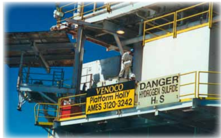
Goodbye (eventually) to Venoco's Platform Holly off the coast of Goleta in state waters, now decommissioned partly due to the oil company's bankruptcy. A celebration of Venoco's demise was recently held at a beer pub in Carpinteria where it has its headquarters, an oil pier and another offshore platform, in anticipation of recovering 45 acres of bluff-top lands. (Photo by Robert Bernstein)
