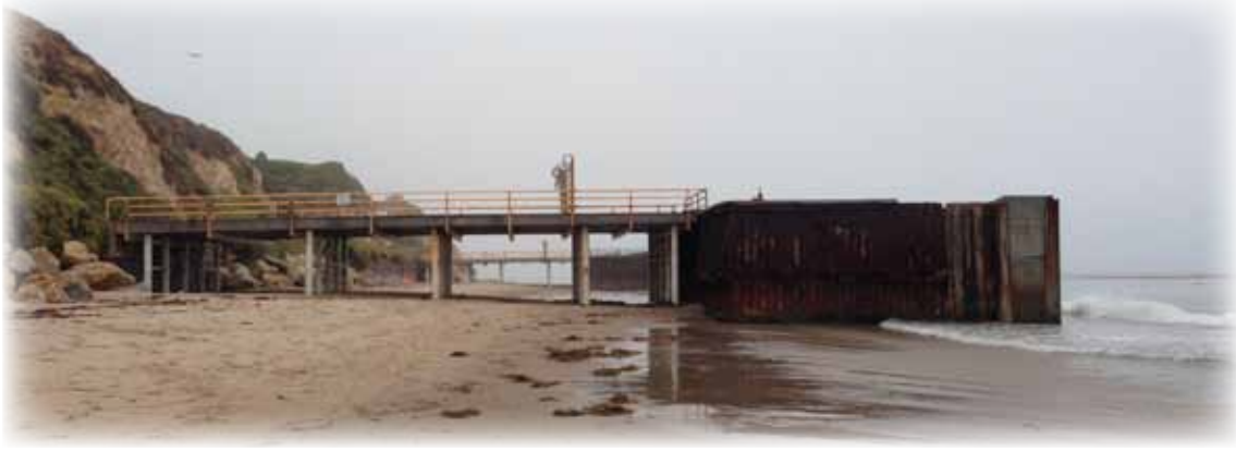
Pier 421 on Ellwood Beach should be gone within a year due to California State Lands working to dismantle the region's old and crumbling oil infrastructure. (Photo by Katie Davis)
