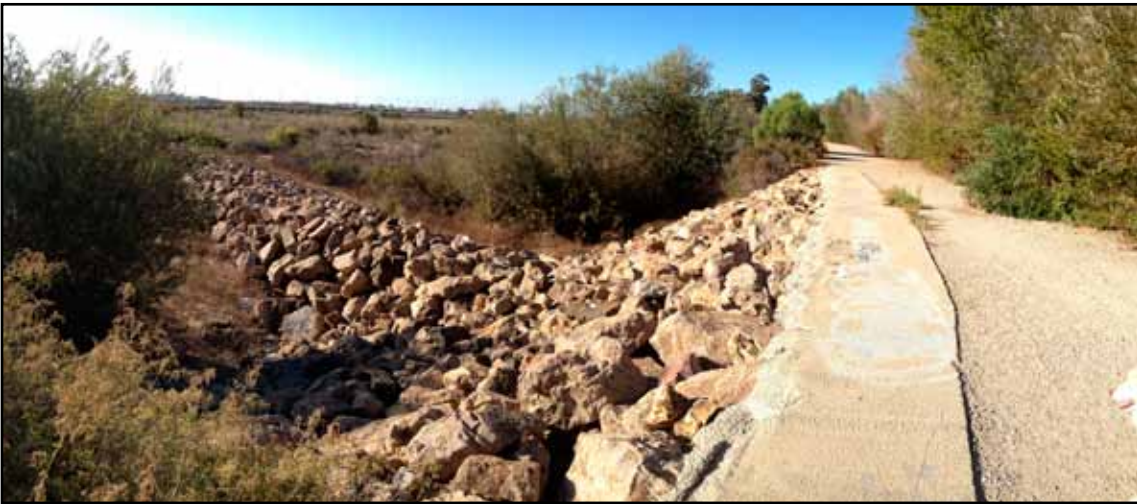
Here's a local example of some attempt to ensure rainfall is recharged into the ground via some green flood control measures on the north bank of the Santa Clara River. (Photo contributed)
