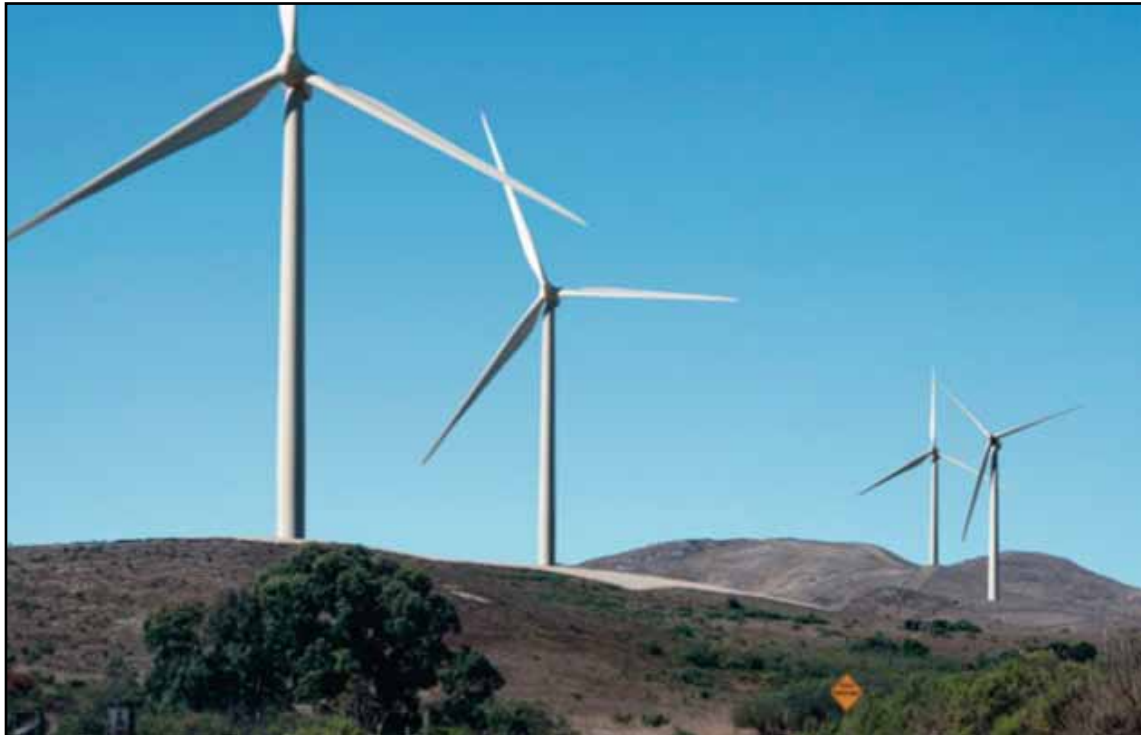
Strauss wind project designed to power equivalent of 45,000 homes, generating $40 million in taxes over 30 years. This renewable energy reduces up to 200,000 metric tons of CO2 annually via 30 wind turbines up to 492 feet tall. Location over 2,970 acres east and northeast of Lompoc. (Source: SB County)
