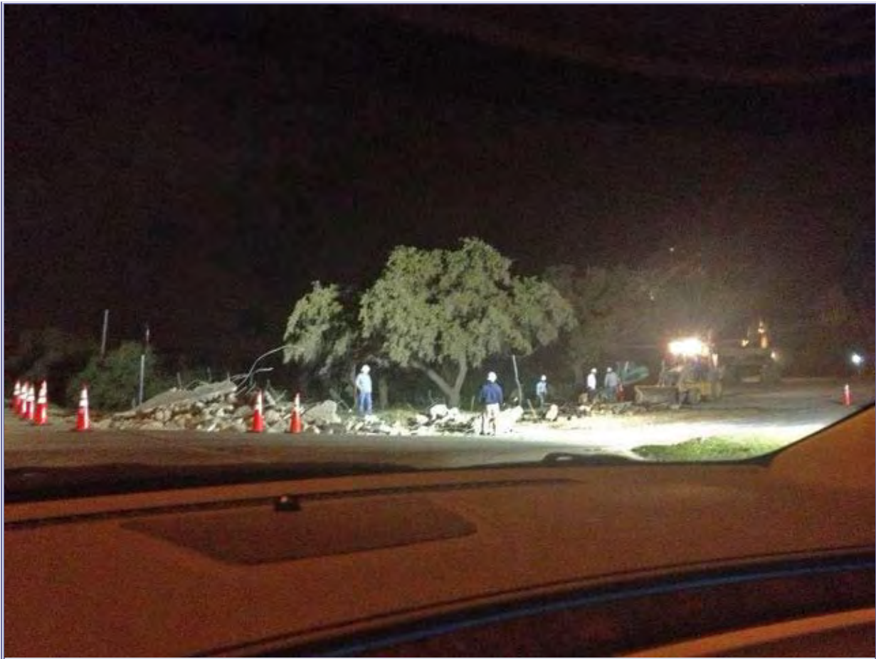
Friday night construction work at entrance to Vulcan Material plant
