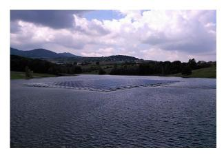
Putting systems on water instead of land is catching on. Attach solar panels to rafts that float on top of the water in lakes. Some of the benefits:
