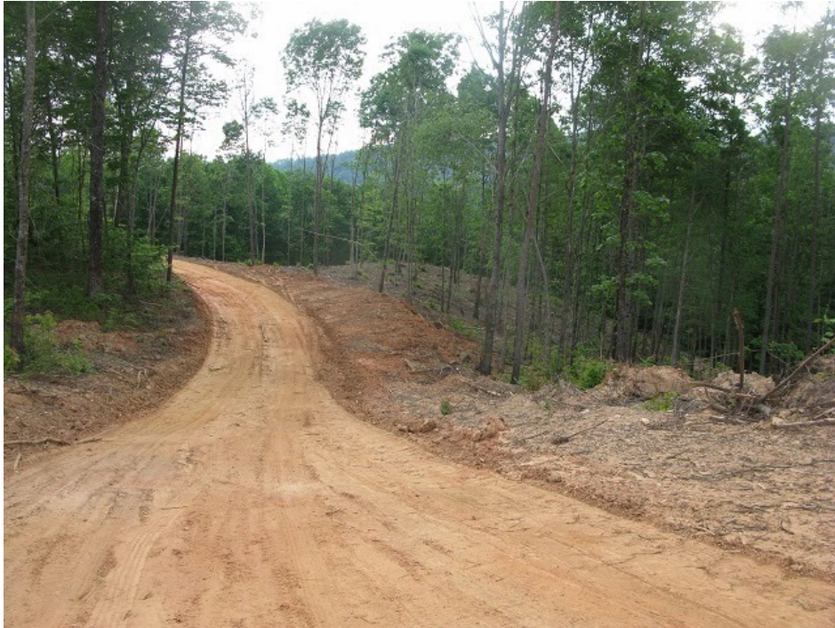
"Temporary" Road up the East ridge of Brawley Mountain project area.
