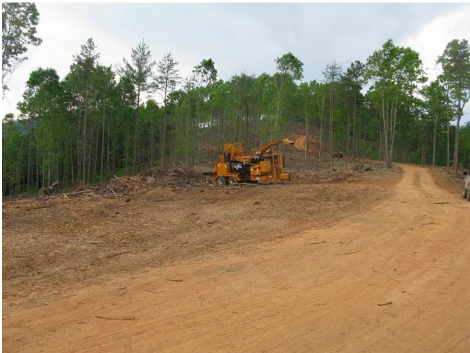
Chipper set up on East ridge.
