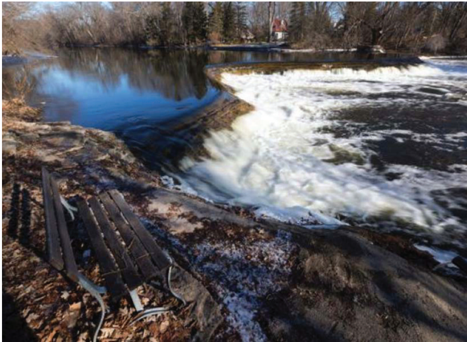
Plans for the Kletzsch Park dam in Glendale have gone back to the drawing board with an eye toward preserving trees and maintaining the character of the river's west bank.
