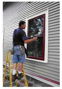
Storm windows with Low-E glass installed over original restored windows, creating a well-sealed secondary glazing
