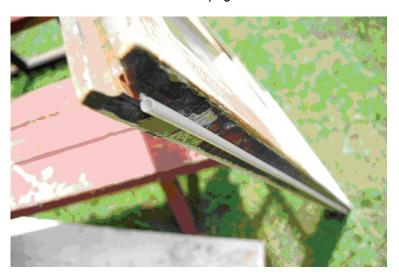
IMAGE 2: Silicone tube seals in kerf in the head of the upper sash, at the meeting rail of the lower sash, and at the sill of the lower sash.
