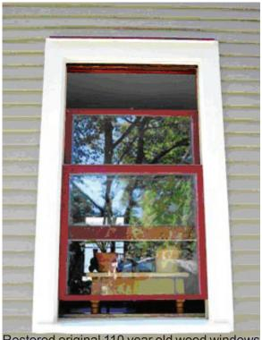
Restored original 110 year old wood windows with draught proofing - 66% air leakage reduction
