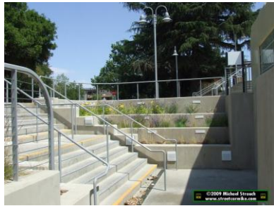
Pedestrian-bike passageway under train tracks – Palo Alto
