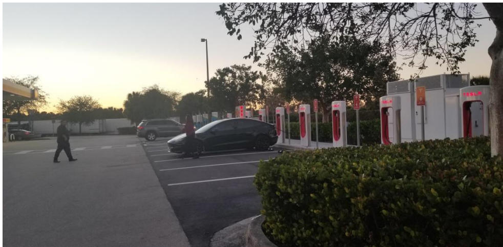
Figure 19 Plug in charging station at Florida Turnpike Lake Worth Service Plaza on the east side looking west
