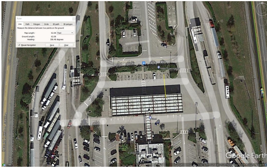
Figure 18 BEV charging station at the Florida Turnpike Lake Worth service plaza Picture source: Google Earth
