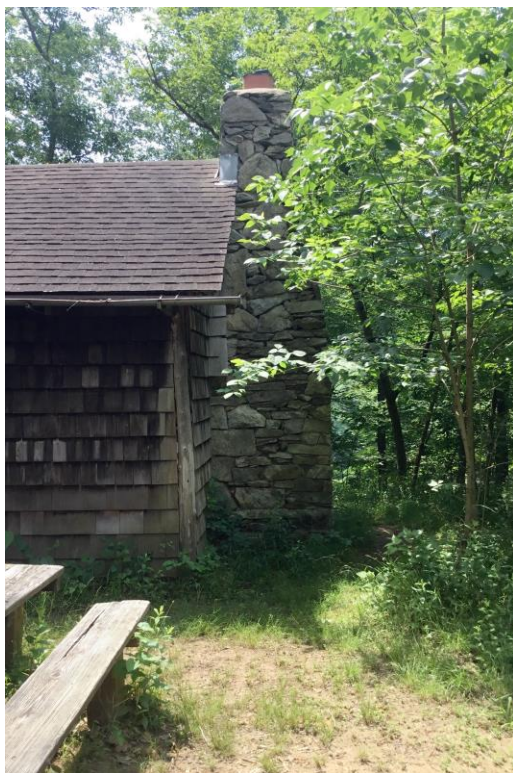
Detail of WBFC cabin chimney stack on west elevation, looking south.
