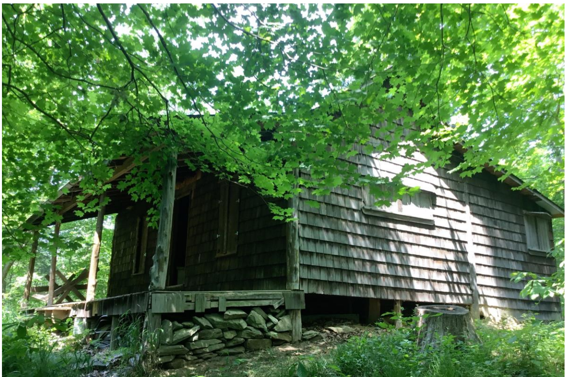
WBFC cabin, northeast oblique.
