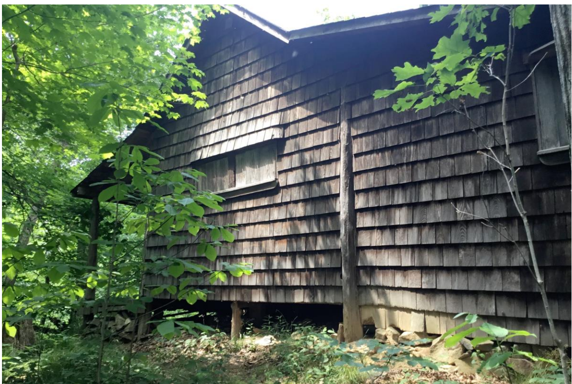
WBFC cabin, east elevation.
