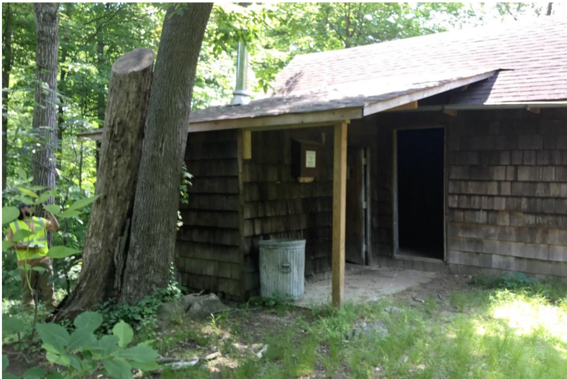
WBFC cabin kitchen projection, north elevation, looking southeast.
