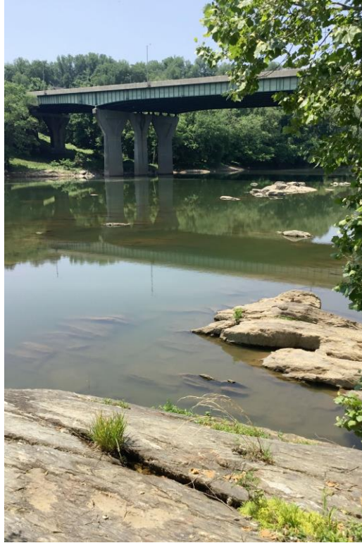
Plummers Island southern shore, looking west towards American Legion Bridge.
