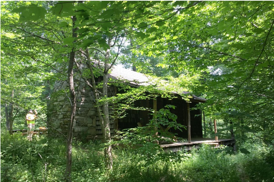
WBFC cabin, southwest oblique.
