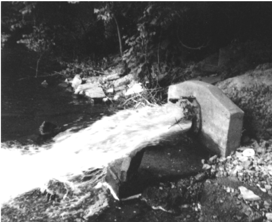
Tyson's discharge pipe empties into Elk River
