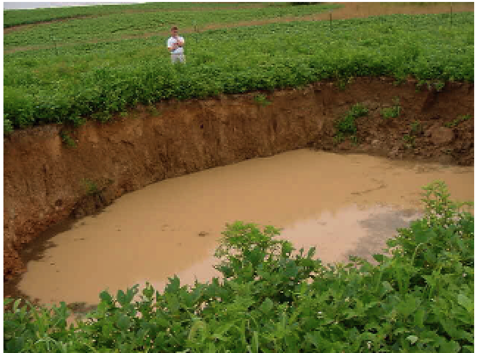
When Kinder-Morgan began exploratory drilling, a hole and cavernous cracks appeared in the soybean field of the neighboring Seabaugh farm.
