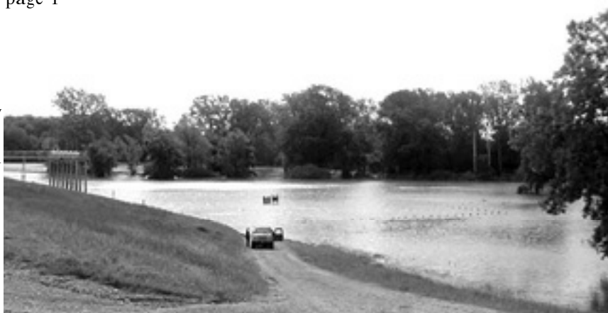
Figure 3. The Swollen Mississippi River backs up through the gap into the New Madrid Floodway. The St. Johns Bayou gravity gate through the set-back levee is at the left.
